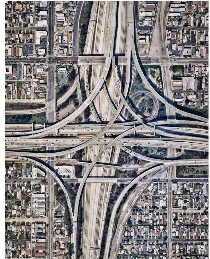
Harry Pregerson Interchange. When interconnection is the problem.
