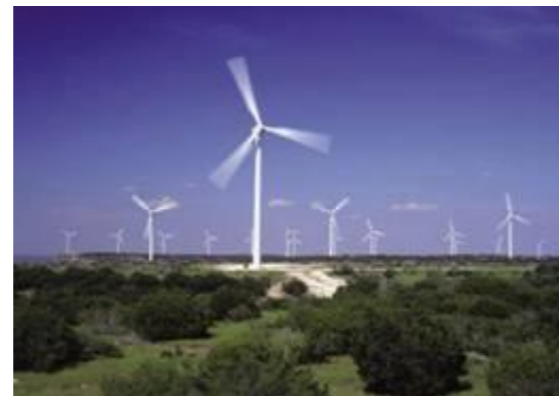
Power generation and distribution
